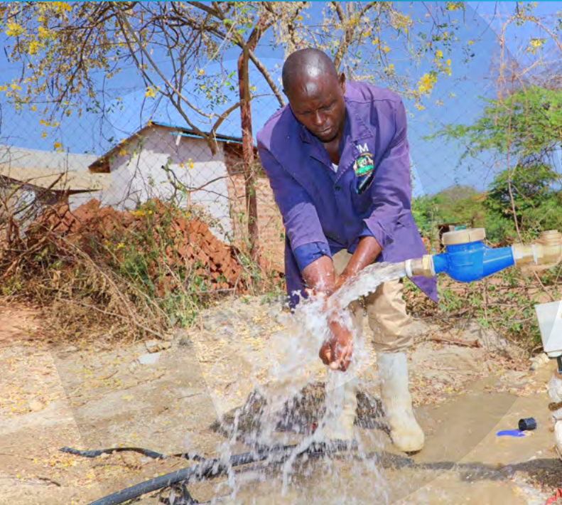
Test-pumping at the Mwingi Slaughterhouse borehole
