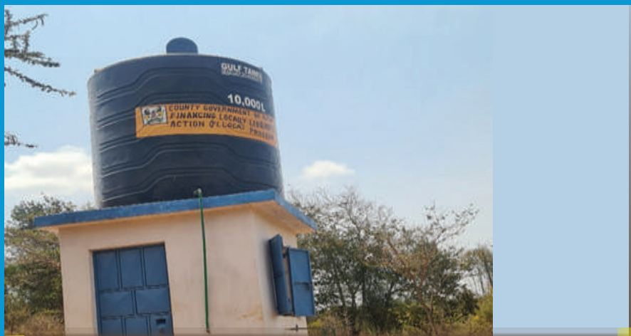
Water Kiosk for the Pipeline extension at Tulia Kangenge, Mutonguni Ward, Kitui West
